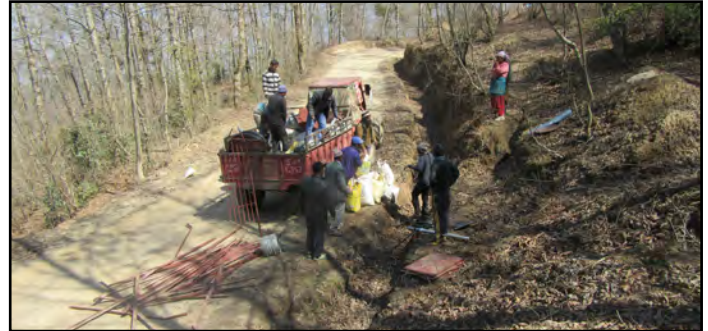
Transporting water system materials on mountain roads (file photo).
